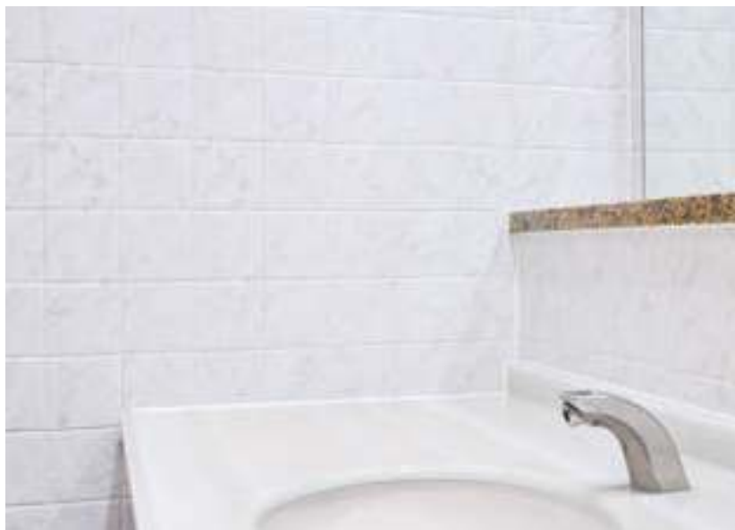
Restroom refurbishment / ST-024TIL
